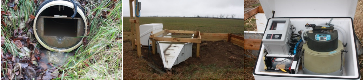
Figure 2. Example of EOF monitoring equipment in Ohio (photos by Tom Bruulsema).
